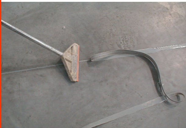
Quick Joint 85 protects concrete joint edges from wheel pressure.
